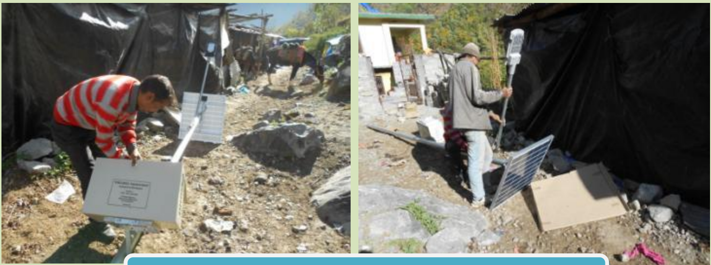
Technical Staff Assembling the Solar Street Lights Equipments
